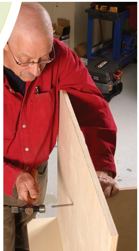
Transfer the pilot-hole locations. With the two panels aligned and held in place, slide a center punch through the outer panel and tap it to mark locations for the pilot holes. Disassemble the parts and drill the holes.
